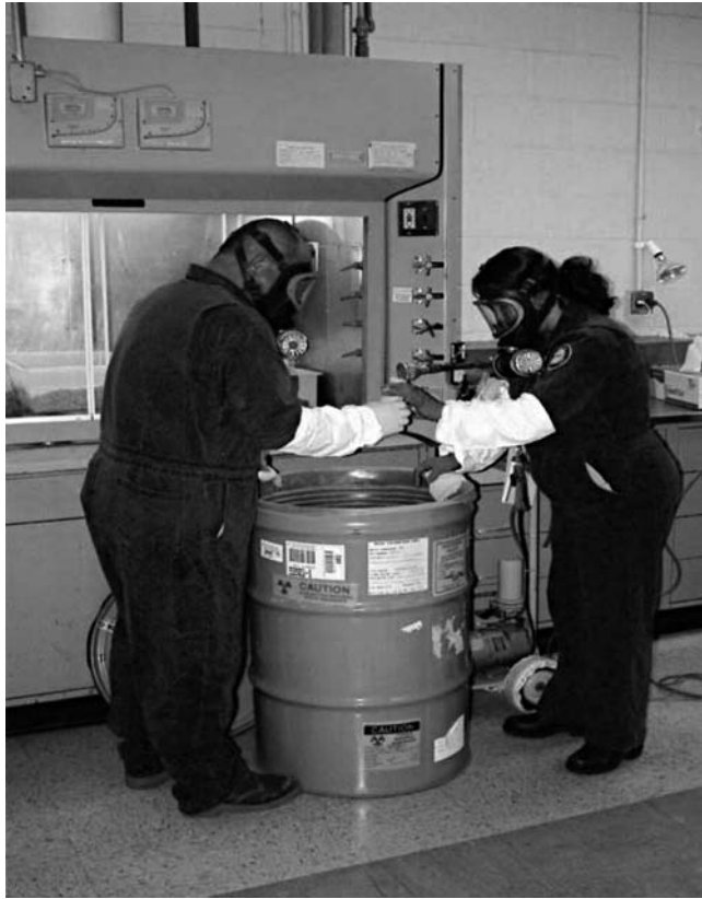
FIGURE 14.8 D&D work in front of equipment with PPE.
