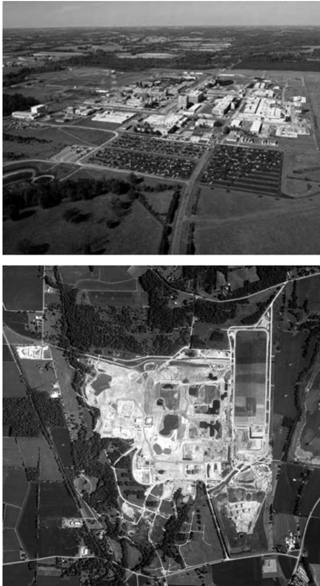
FIGURE 14.1 Aerial view of the Fernald, Ohio Site before cleanup (1987) and after cleanup (2006).
