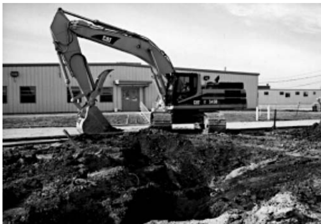
FIGURE 14.17 Typical structures for mobile lab or shower facilities.
